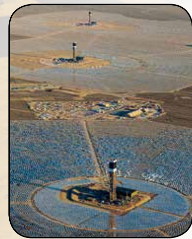
Ivanpah - Plant of the year 2014
